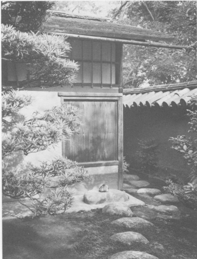
Small entrance ( nijiri-guchi ) of tea-house Shinju-an in the Daitoku-ji Temple, Kyoto. Photograph by Yukio Futagawa.
